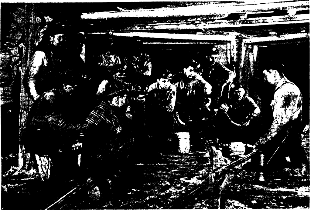
Miners in the Willow Grove Mine of St. Clairsville, Ohio, discussing safety measures. Note the electric lamps attached to the miners' caps. Each lamp is connected by means of a cable to a battery carried on the belt.
