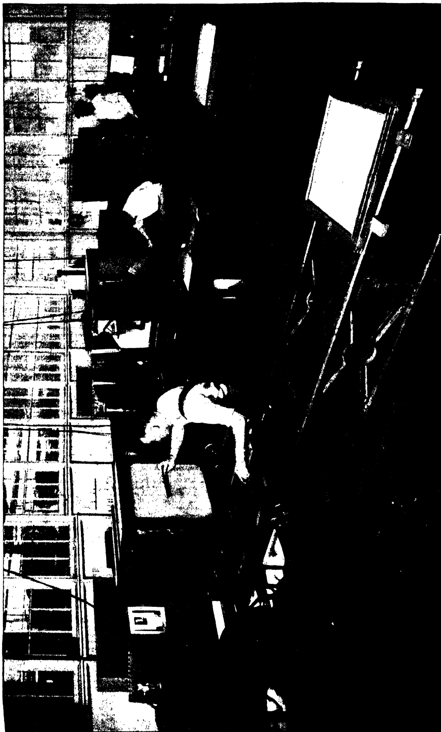
Courtesy, Haddon Craftsmen This illustration shows us how halftone cuts are made. The photograph, or "original" as it is called, can be seen on the left with the strong light shining on it. It is having its picture taken by a special camera. In front of the photographic plate has been placed a fine glass screen, so fine that the copper plate will be covered with tiny dots. Because of these dots, the reproduction is printed in tones of gray, like this one, and hence the name, "halftone."
