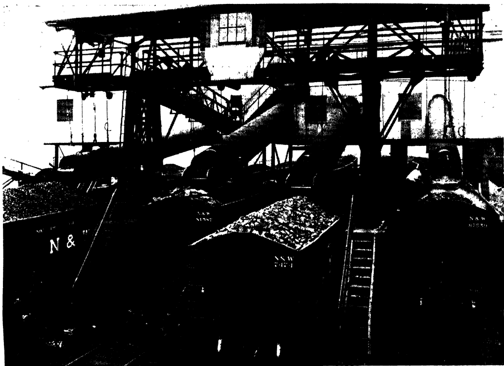
After the coal has been cleaned and graded, it passes into huge bins, which are set over railroad tracks. From these bins the coal slides down sloping chutes into open freight cars waiting on the tracks below. Most of the coal that is mined in North America is carried to market in freight cars like those shown in the above picture.
