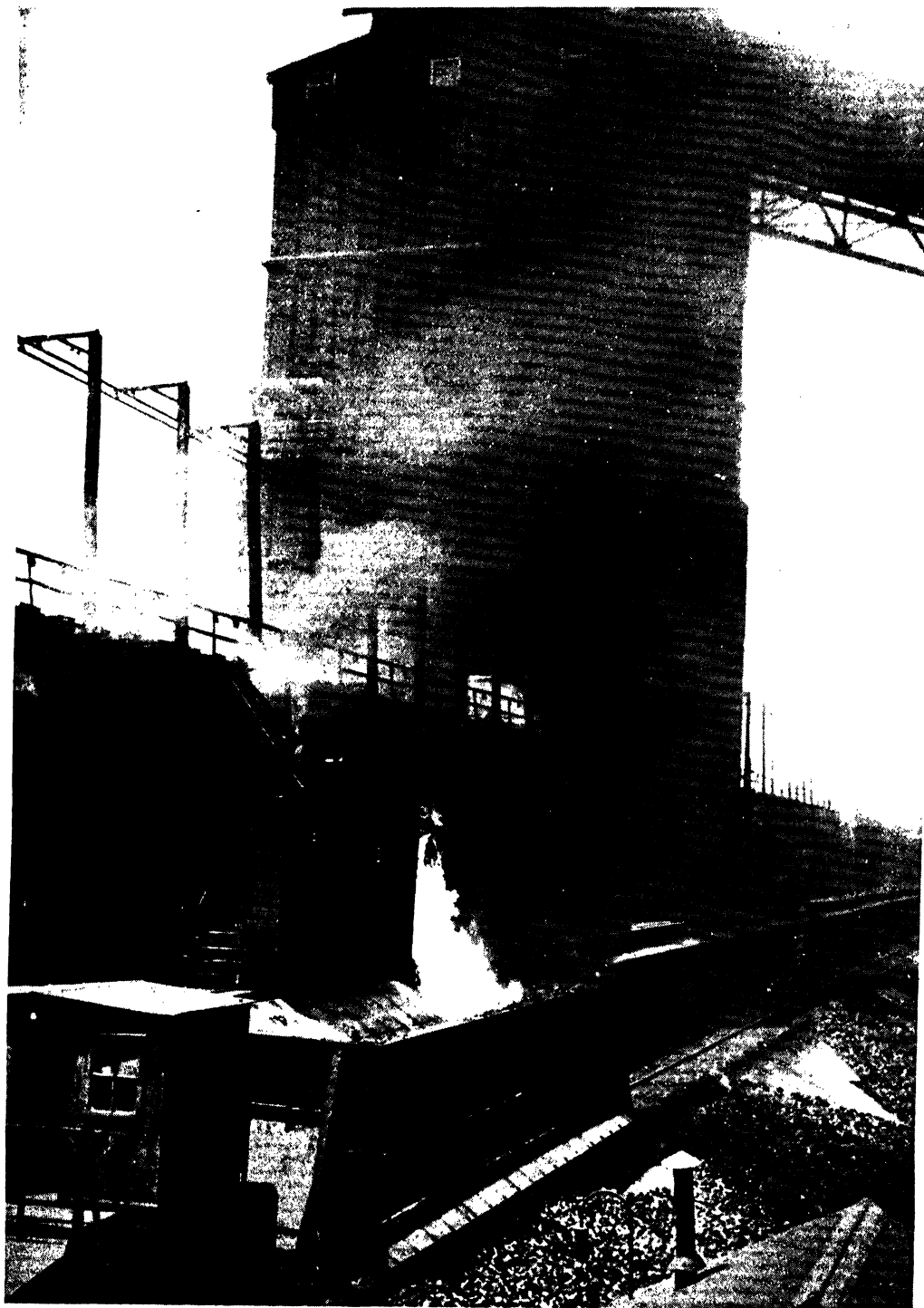
This striking picture shows bituminous coal being converted into coke in a battery of by-product ovens. These ovens, as the name indicates, are specially designed to save the valuable by-products of the coking process.
