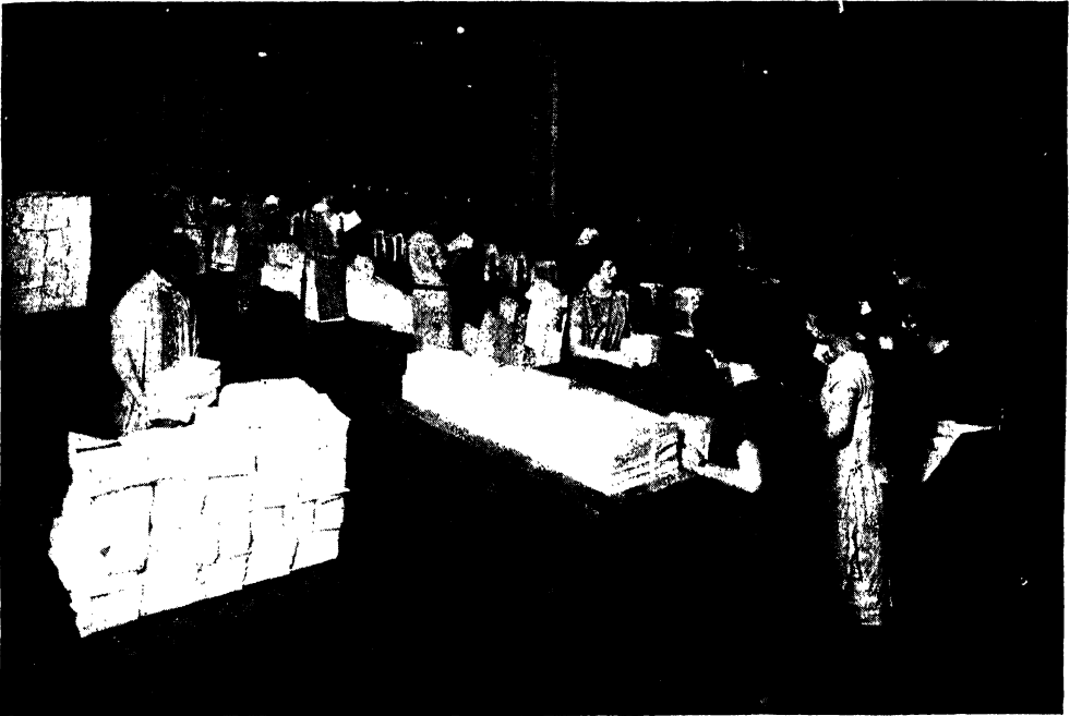
The girls in the background are placing the sections of a book into a gathering machine.
