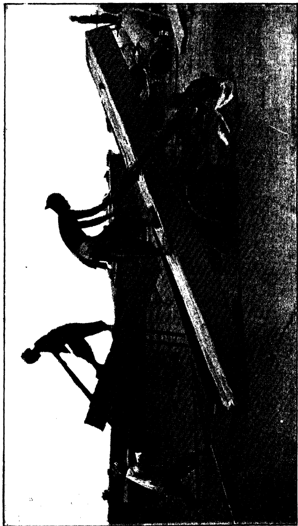
CARPENTERS SAWING LARGE TIMBER.
