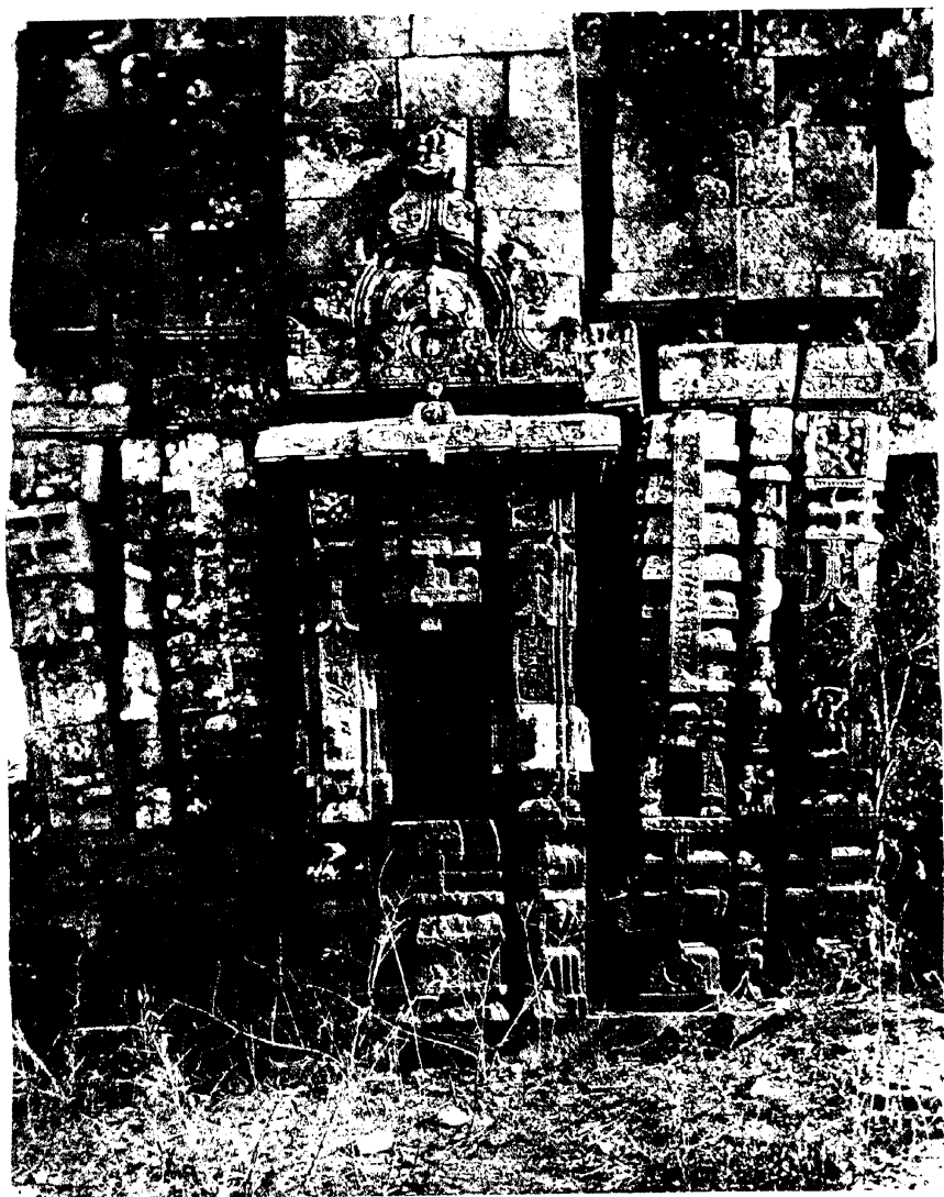
Bāra consisting of pābhāga , fāṅgha and baranda in a ruined Temple near Kotitirtha, Bhubaneśwar
