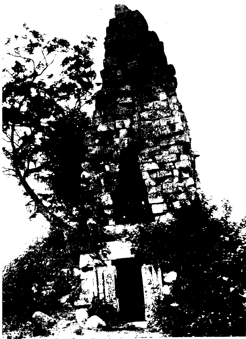
Corbelled arch above the lintel in a ruined temple near Rameśwar, Bhubaneśwar
