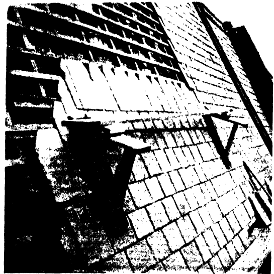
FIG. 15. SLATE BATTENS AND COUNTER BATTENS IN SLATED ROOF
