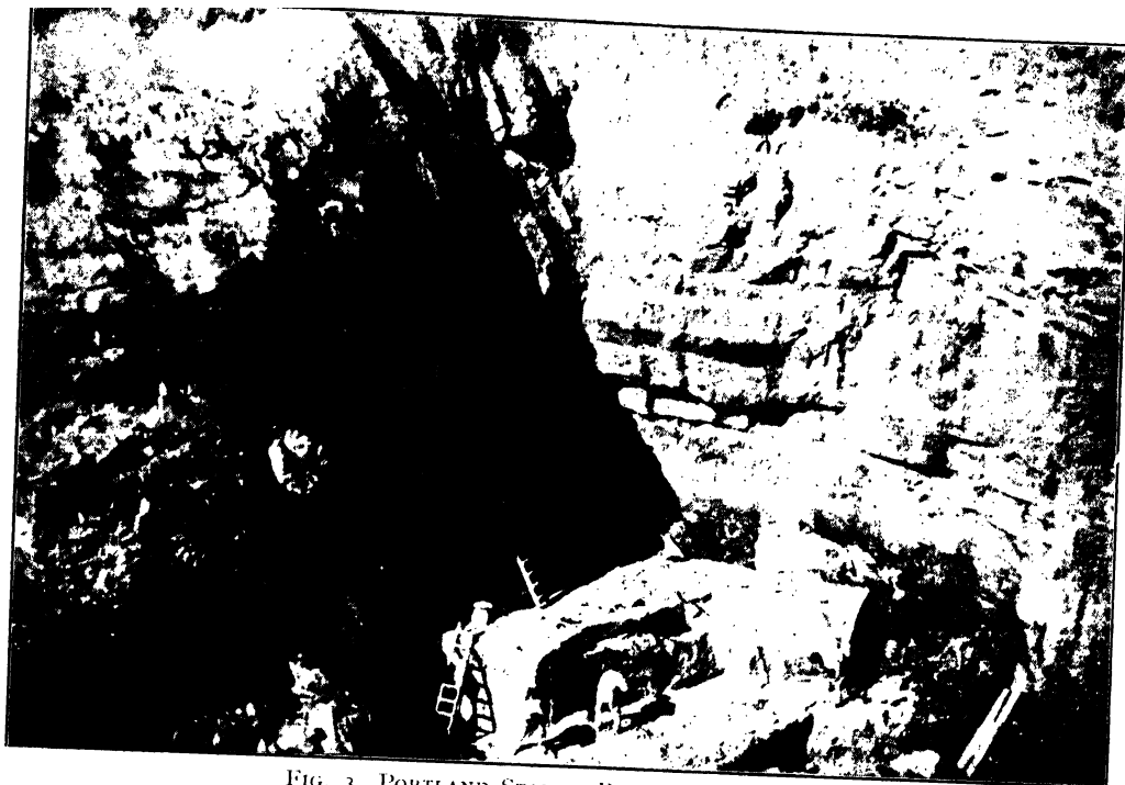
FIG. 3. PORTLAND STONE: PERRYFIELD QUARRY Showing depth of stone compared with the amount of waste or rubble By kind permission of The Bath & Portland Stone Firms, Ltd., Bath
