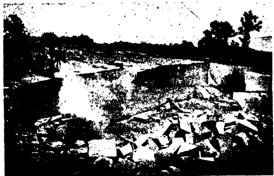
FIG. 9. WINNSBORO BLUE GRANITE, RION, SOUTH CAROLINA, DRILLING FOR BLASTING AT QUARRY FACE Position of latest blast can be seen on the right
