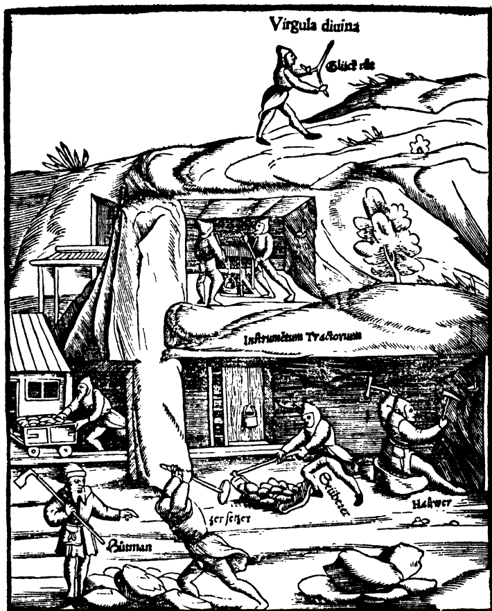
Fig. 19. A sixteenth-century minehead railway. Note also the crude winding by winch in this case.
