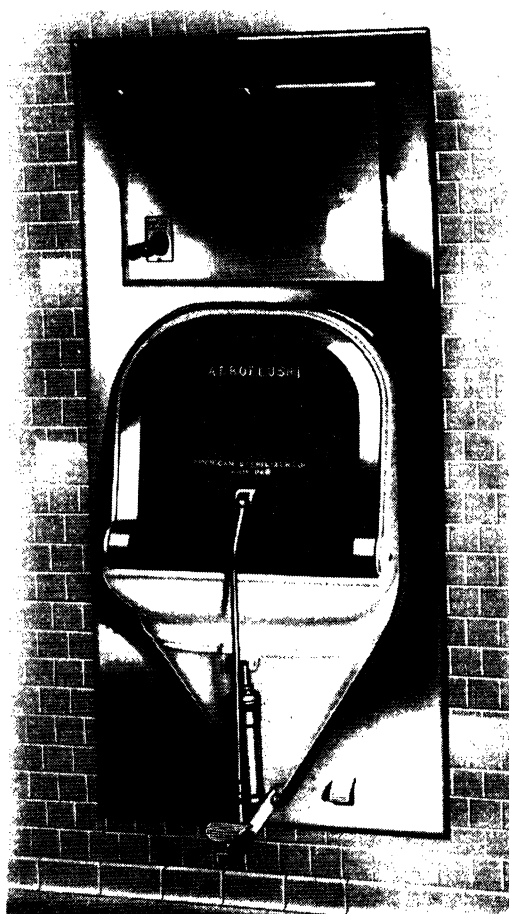
FIG. 83. Built-in type bedpan and urinal washer and sterilizer. This type occupies slightly less floor space, performs exactly the same as the wall suspended type.
